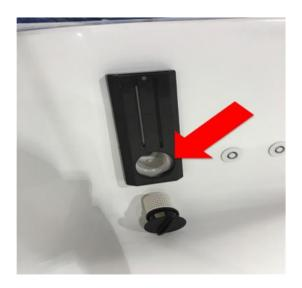
2) Make sure the nut on the filter is loose, allowing air to move through the system. See below
